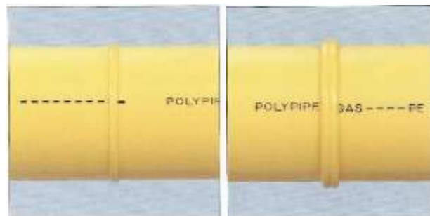
Melt bead too small due to insufficient heat time.
